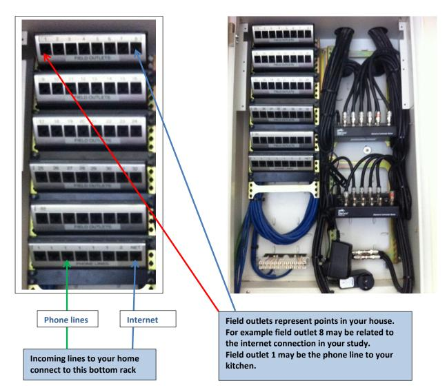
The example to the right is a different design but the same principle. In this example the incoming internet has been connected to the field outlet in your house that is numbered as four.
